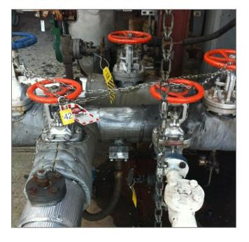
Sensor in byPass line with flushing ports
